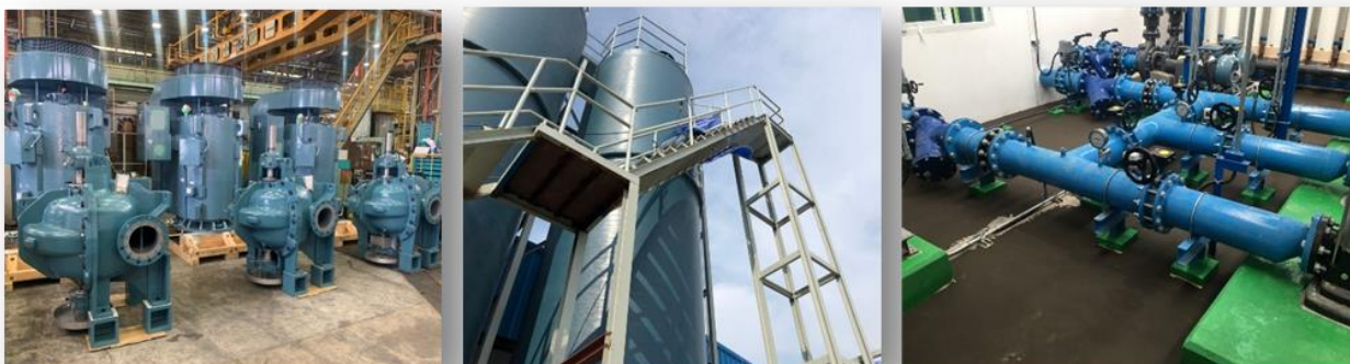
Water management facility
