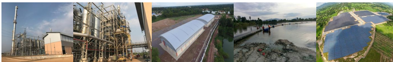
Project of Industrial Waste Power Plant
