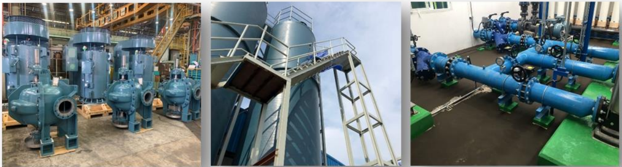
Water management facility
