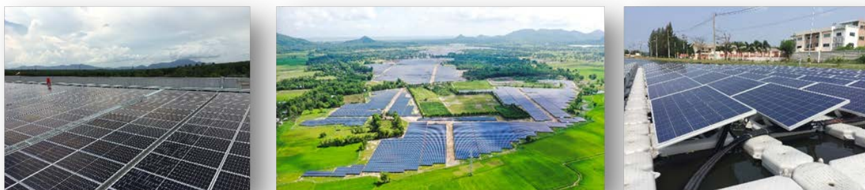
Solar Plant – installed on rooftop, on ground, and floating on water (from left to right)
