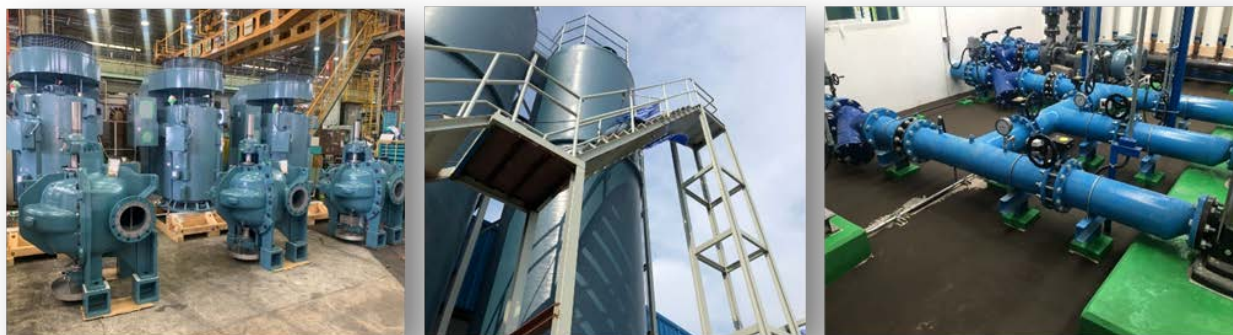
Water management facility
