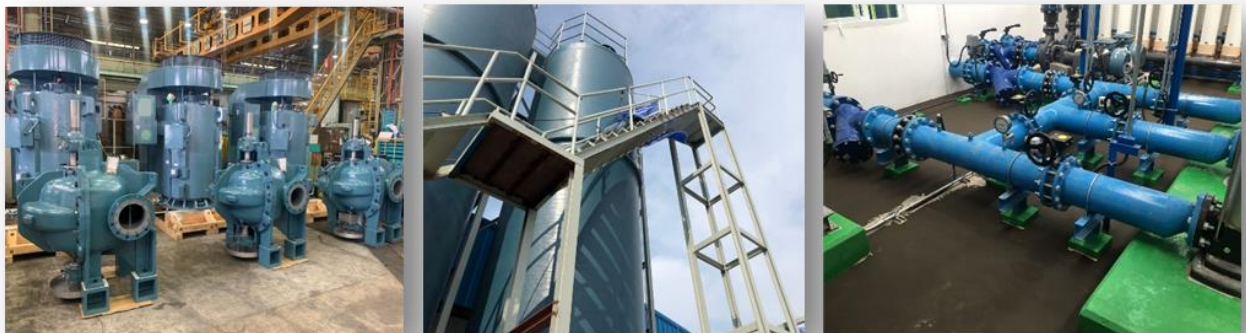
Water management facility
