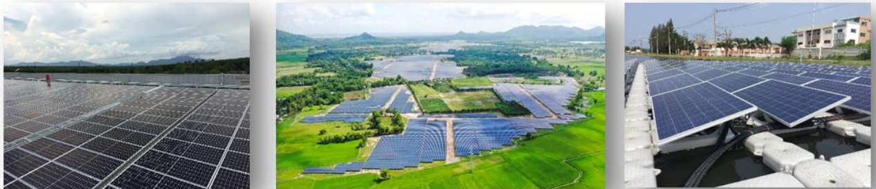
Solar Plant – installed on rooftop, on ground, and floating on water (from left to right)
